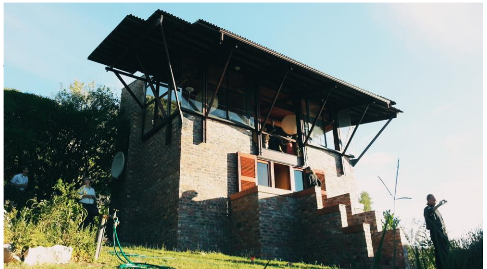
Figure 10. House Uytendogaardt, Roelof Uytendogaardt, 1993. View of the entrance and upstairs living space from the north. Photography by Mallix. Licensed for reuse under creativecommons.org/licenses/by-sa/2.0 .
