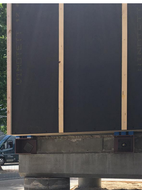
Figure 6–8. Mock-up of Circle House during construction (own photos)
