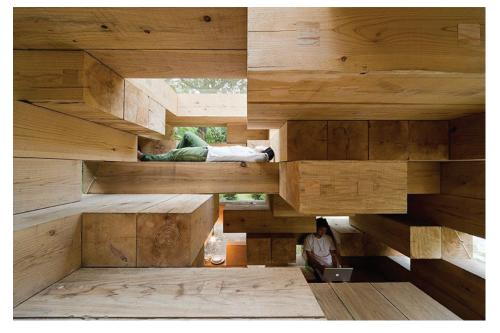
In Norwegian Wild Reindeer Center Pavilion by Snøhetta, the architectural starting point has been the function of the building as a sheltered place for observing the surrounding nature. The outer shell is rigid and cold designed to withstand the harsh climate, while the interior of the building is warm and cozy. Logs of the pavilion are stacked upon each other but also besides each other
