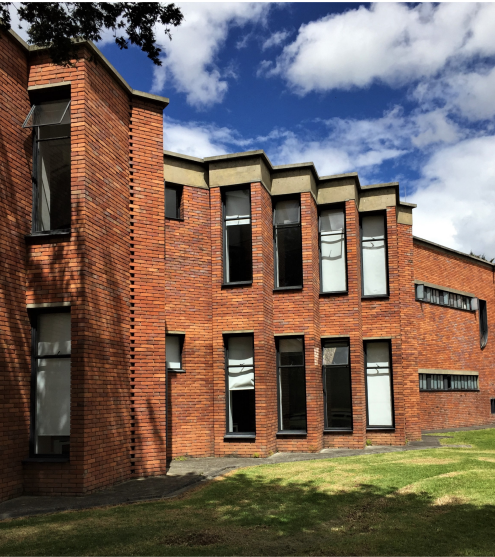
Figure 17. The folded walls of façade of Facultad de Ciencias Económicas. Source: Hernández J. [Photograph]. 2017.
