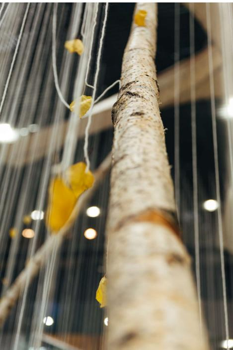
**Figure 14.** Unprocessed tree trunk working as column. Photo credit: Lassi Savola.
