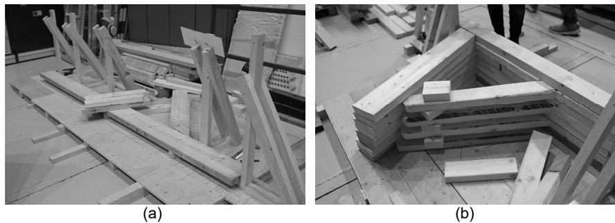
**Figure 14. Making the plaza structure:** (a) the working platform, and (b) the arrangement of timber boards.
