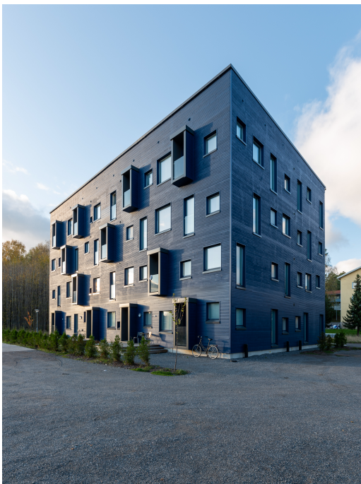
Figure 14. Goliathin Salmi timber apartment building constructed with 2D panel construction method, located in Turku, Finland. Photo courtesy of Vesa Loikas.
