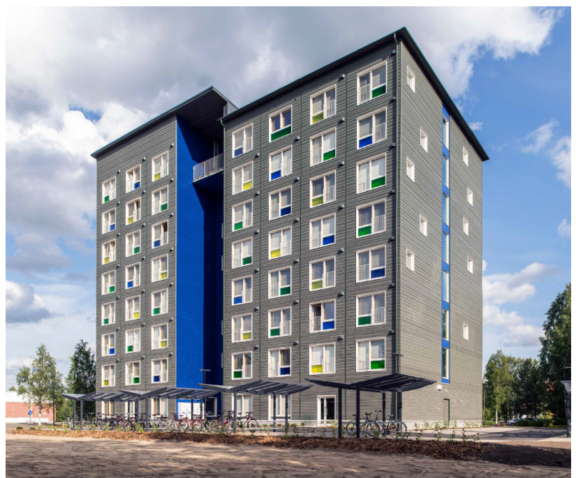
Figure 15. DAS Kelo timber apartment building constructed with 3D volumetric construction method, located in Rovaniemi, Finland. Photo courtesy of Aaro Artto.
