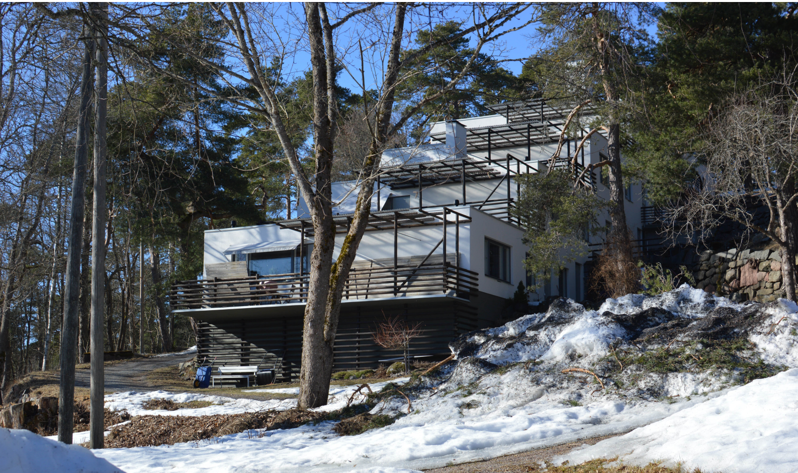
Figure 1. View of Terassitalo from the south. Looking up the steep slope that the house occupies surrounded by both evergreen pines and deciduous trees. Photographed March 21, 2022, 13:41 by Troels Rugbjerg.
