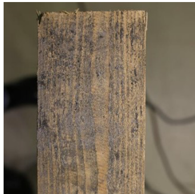
Figure 5. CW Formwork wood – original image
