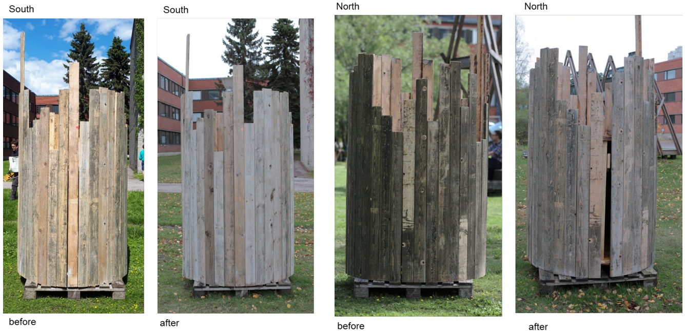
Figure 14. Comparisons of the south and north view of the full scale demonstrator at Aalto University, Otaniemi Campus, Espoo, 60°11'15.7"N 24°49'55.4"E - before and after 4 months of exposure to natural environment June to October 2022.
