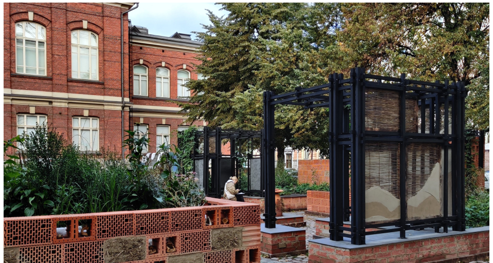
Figure 3a. Alusta Pavilion by architects and doctoral researchers Maiju Suomi and Elina Koivisto, 2022. The pavilion is an experimental research project located in the courtyard between the Museum of Finnish Architecture and Design Museum in Helsinki. The pavilion has served as a platform for empirical research on biodiversity in urban milieu through pollinator-friendly plantation and structures and a multisensory urban space. Suomi and Koivisto also have a mutual professional practice Suomi/Koivisto.
