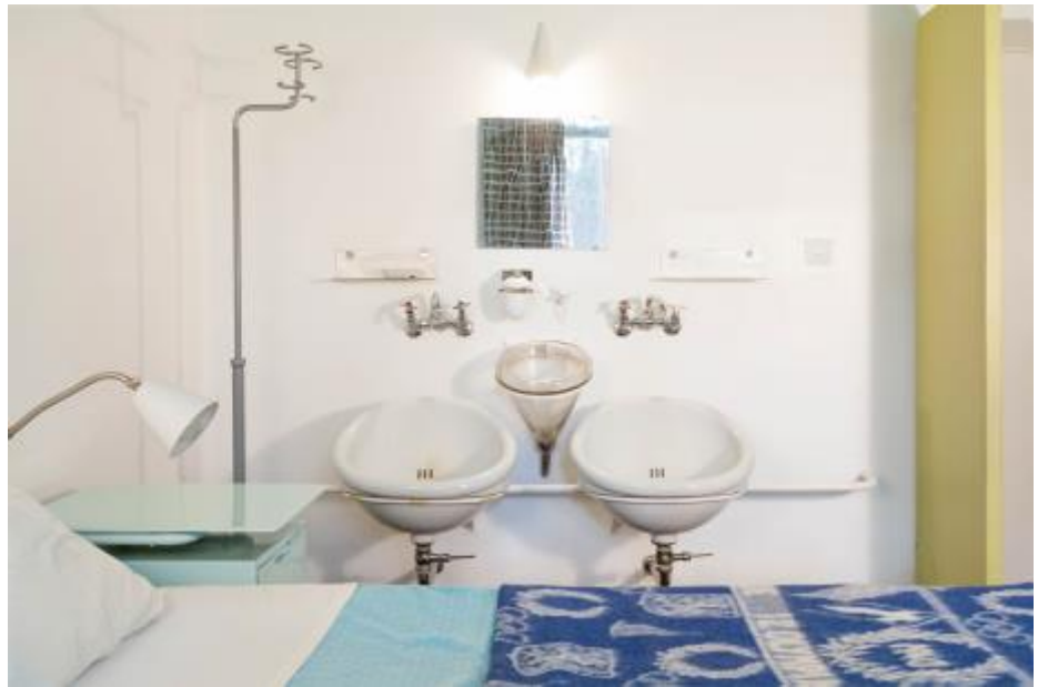
Figure. 1. This photo shows the key hygiene fittings for the patient room. Photo ark-byroo, 2015.
