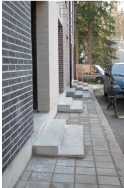
Figures 13 and 14. The incompatibility of street and building execution creates barriers (left). A narrow front yard ensures privacy and allows a sheltered entrance, if correctly dimensioned for wheelchair use. (right) (Kalasatama, Helsinki). Photos Ira Verma.
