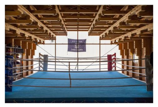
**Figure 20. Use efficient forms for long spans from short pieces.** Although not made of reclaimed timber, this figure illustrates the 5th principle with the corbelled roof structure of Kogakuin University Boxing Club in Tokyo, designed to be built from short low-quality wood (designed by FT Architects, photo in the courtersy of Jonas Aarre Sommarset).
