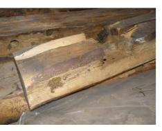
Figure 13. Reduction of crosssection. A notch in a log.
