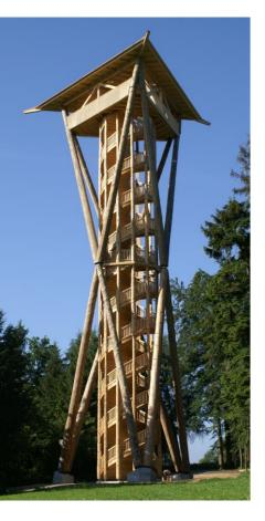
Figure 4. Wood is lightweight and linear, i.e. a tectonic material. A lookout tower in Wil, Switzerland, designed by Julius Natterer. Photo by Touristinforwil, downloaded from Wikimedia Commons and published under the license CC-BY-SA 3.0.
