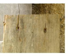
Figure 15. Cracking and nail holes at the end of a floorboard.
