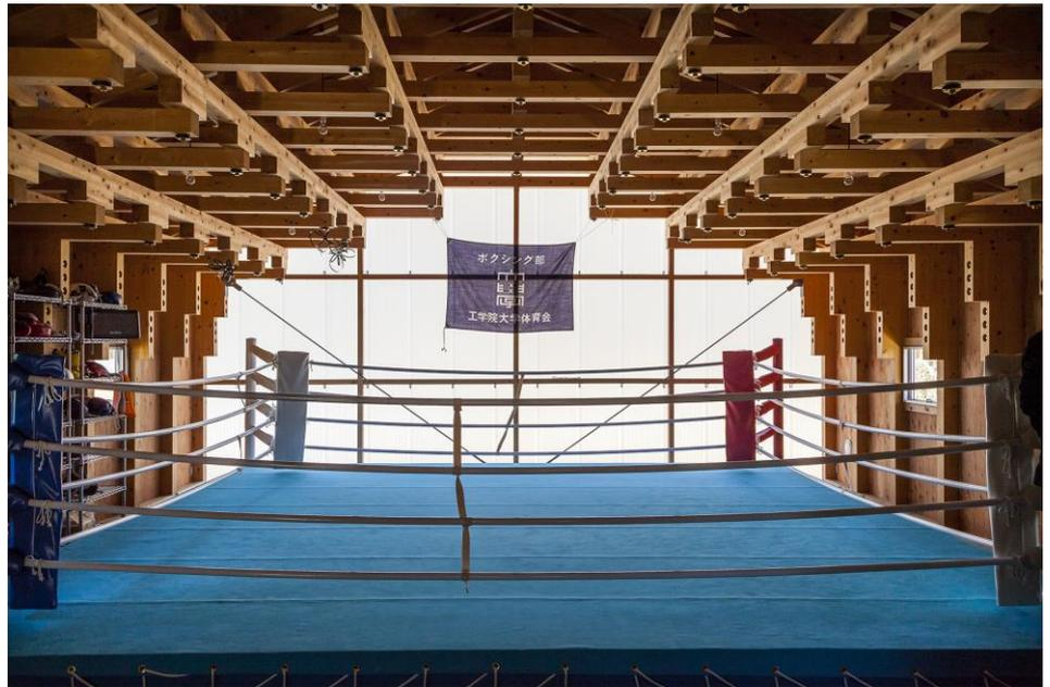
**Figure 20. Use efficient forms for long spans from short pieces.** Although not made of reclaimed timber, this figure illustrates the 5th principle with the corbelled roof structure of Kogakuin University Boxing Club in Tokyo, designed to be built from short low-quality wood (designed by FT Architects, photo in the courtesy of Jonas Aarre Sommarset).
