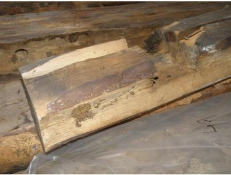
**Figure 13. Reduction of cross-section.** A notch in a log.
