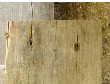
**Figure 15. Cracking and nail holes** at the end of a floorboard.
