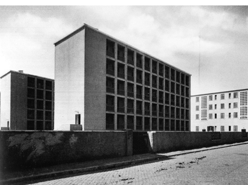
Figure 12. A balcony-access building type (casa a ballatoio) in Block 2 along Via Ostuni, Quarticciolo. Photo: Nicolini (2010, 69).C
