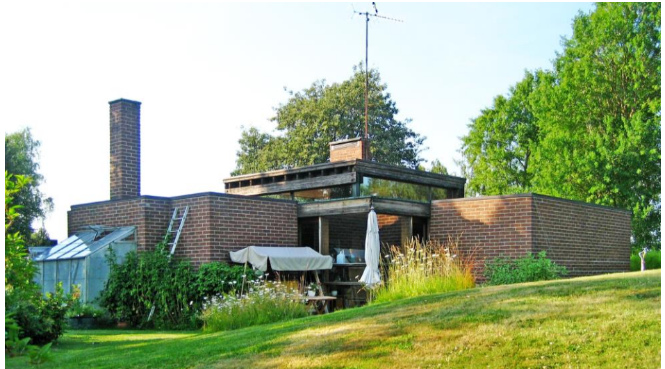
Figure 4. Villa Norrköping, Sverre Fehn, 1964. The view from the south.
