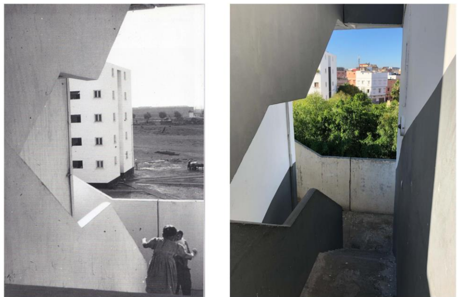
Figure 16. 'Inside the Semiramis building'. Comparison between photos of 1951 (left) and 2018 (right. Photo by the author). Left image in: Avermaete, T. & Casciato, M. 2014. Casablanca Chandigarh. Bilans d'Une Modernisation . Chicago: University of Chicago Press, pp. 291.
