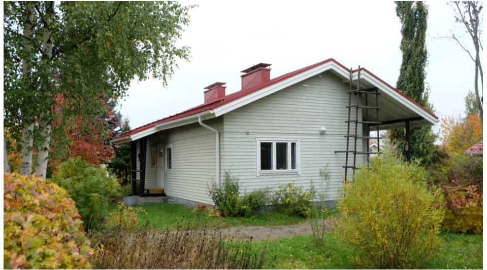
Figure 1. Housing for ex-service men, Alvar Aalto, 1941. View from Saviniementie. Author.
