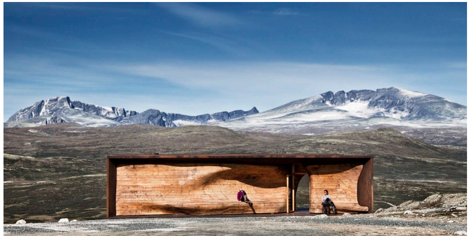
Figure 12. Free shaped log structure is visible in the façades of Norwegian Wild Reindeer Center Pavilion. (Image courtesy of Ketil Jacobsen)
