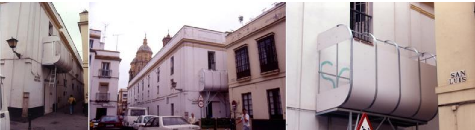
Figure 1. Subversive strategies of urban occupation: scaffolding. Recetas Urbanas (Urban Prescriptions) by Santiago Cirugeda, Seville, 1998. Image source: www.recetasurbanas.net .
