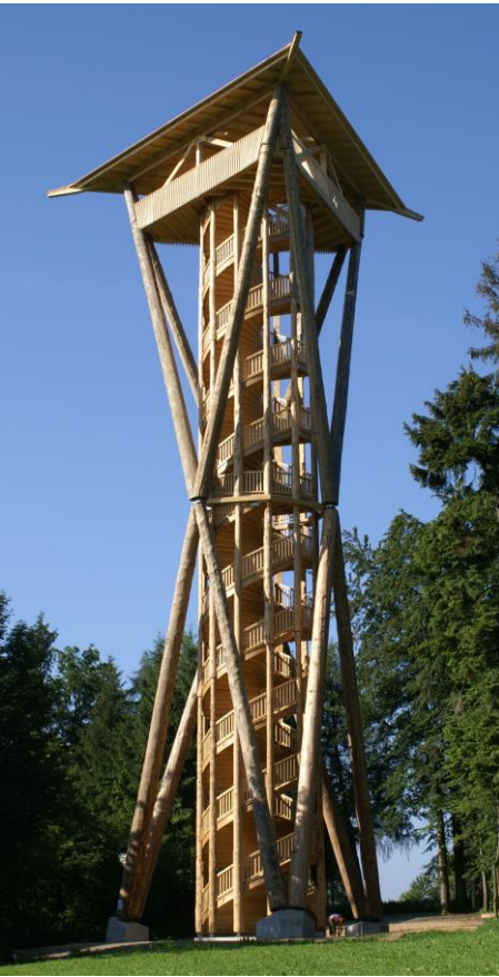
Figure 4. Wood is lightweight and linear , i.e. a tectonic material. A lookout tower in Wil, Switzerland, designed by Julius Natterer. Photo by Touristinformwil, downloaded from Wikimedia Commons and published under the license CC-BY-SA 3.0.
