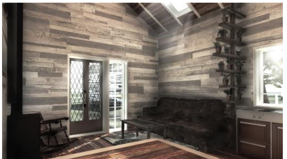
Figure 23. Select the application according to the properties. Interior cladding made of short boards that would otherwise be practically useless (design and image by Razvan Iov).
