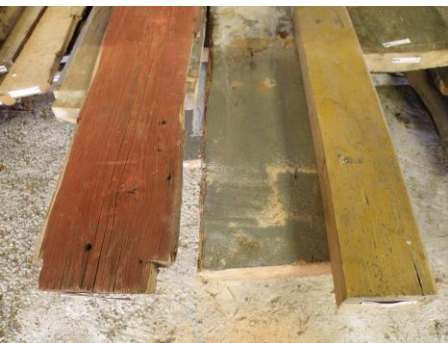
Figure 9. Painted members, traditional red ochre (left) and more modern paints (middle and right).
