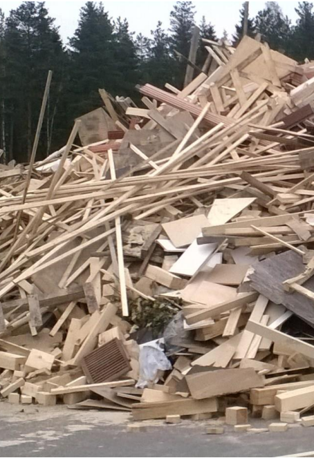
Figure 2. Demolished wood in an ordinary sorting facility: inconsistent in quantity, quality, dimensions, availability and compatibility. Photo courtesy of Paavo Huuhka.
