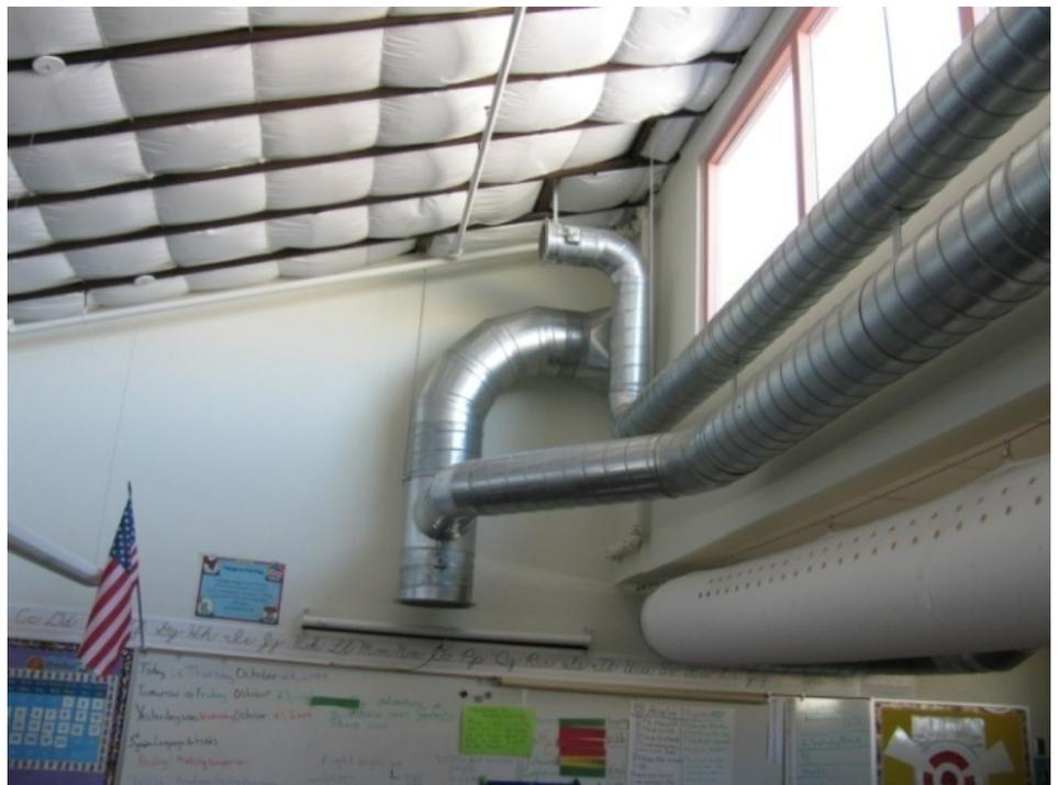
**Figure 8. The typical image of HVAC system ductwork and ceiling insulation exposed in every classroom at Davidson Elementary School.**
