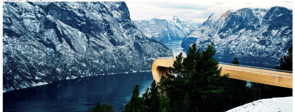
Figure 7. Stegastein viewing platform (2006) by Todd Saunders and Tommie Wilhelmsen. The concept of Stegastein is expressive and iconic but still minimalistic and respecting the surrounding nature. © Nils Vik
