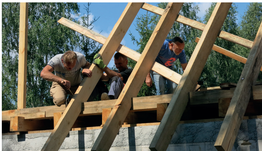
Figure 4. The pottery school being built, 2022 (photo: E. Klekot).
