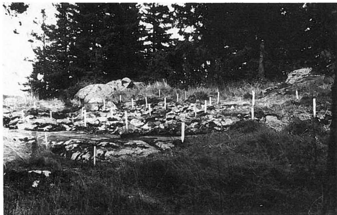
Fig. 3. Paaso: Building foundations.
