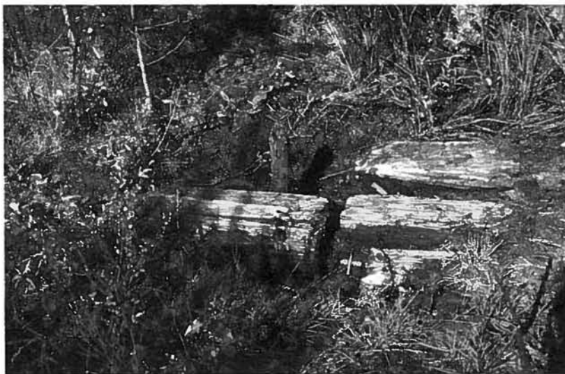
Fig. 5. The construction of the causeway in the bog of Haukivahonsuo.
