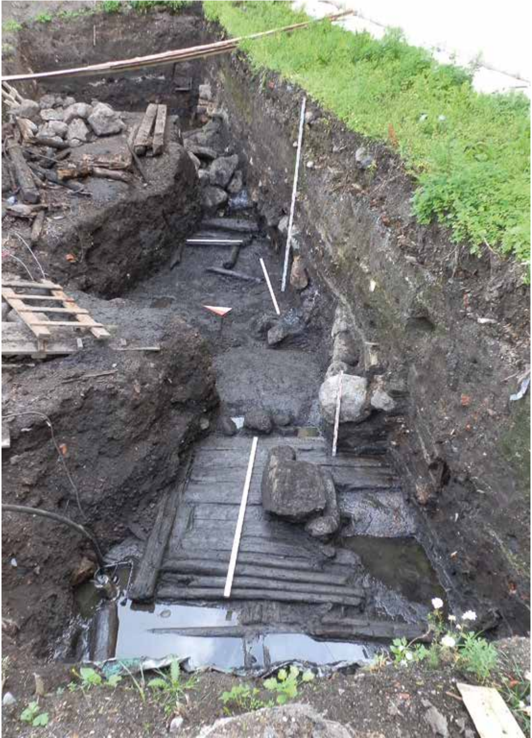
Figure 7. Excavation Area of 2012 at 8 Ul. Vyborgskaya street. The foundation of the building dated to the second half of the 15 th century. Photo A. Saksa.
