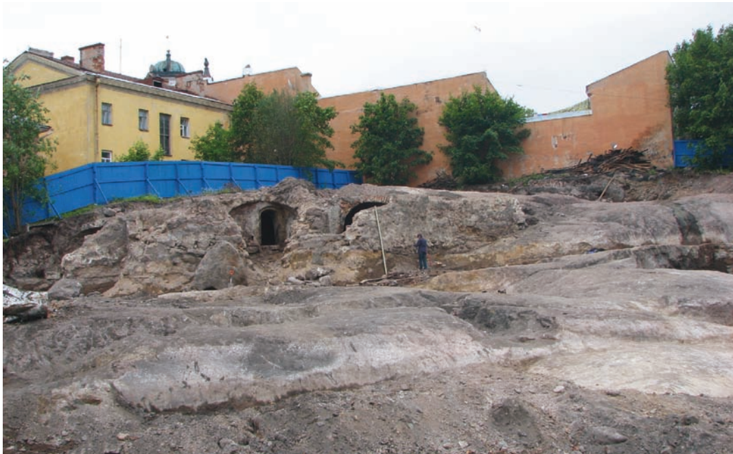
Figure 7. The survey at Ul. Krasnoflotskaya street in 2007. Nothing from the stone cellars had been visible on the surface. Note the topography of the bedrock. The photo was taken from the east by A. Saksa.
