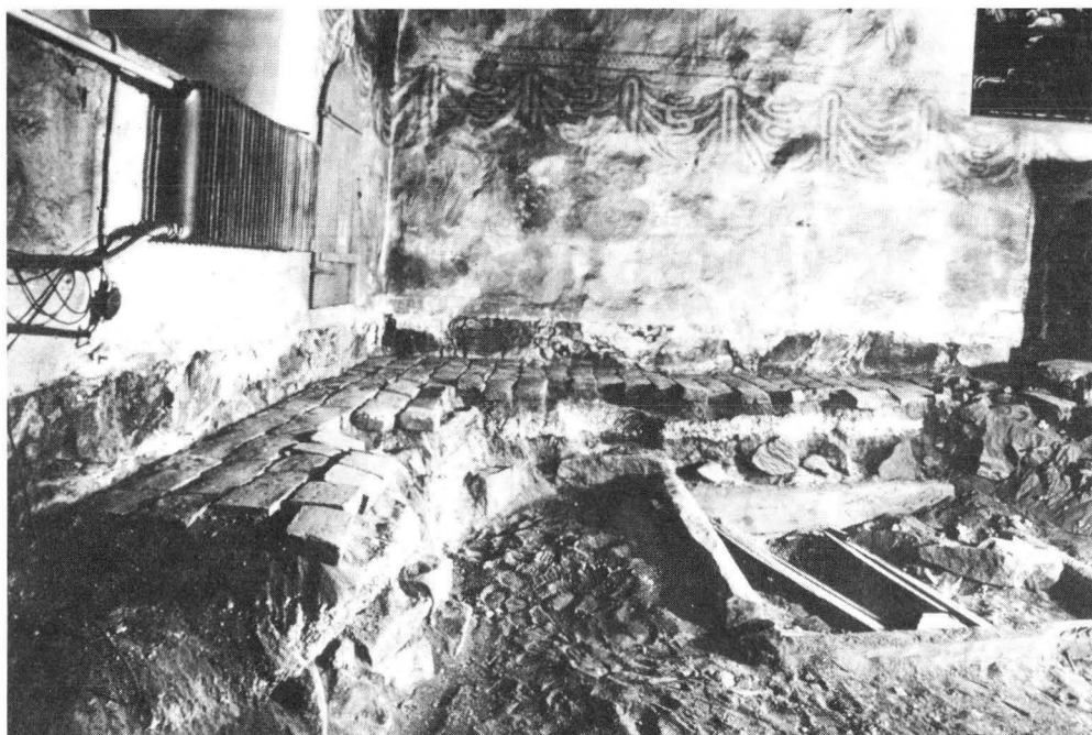
Fig. 2. Part of the medieval brick floor in the northern part of the choir of Espoo church, viewed from the west. Note the thick underlying structure. Archives of the Department of Monuments and Sites, National Board of Antiquities, Helsinki. Photo Matti Huuhka.
