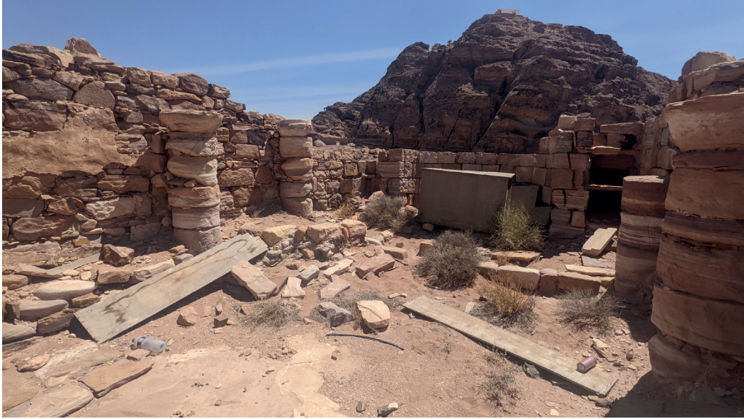
Figure 19. A view of the Jabal Haroun chapel taken in August 2022. Wooden shelters built to protect the most vulnerable parts were broken and the structures themselves badly eroded. The plywood cover protecting the altar box had been thrown aside but is here restored back in place. Bushes have also taken root inside the building. Photo: Antti Lahelma.
