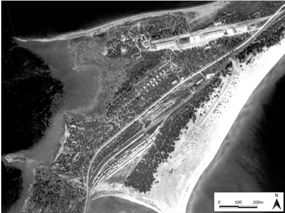
Photo 138. Aerial photo of the area of Deutsches Lager Hanko taken on 27 May 1950. Most of the buildings of the camp have been dismantled. Original photo edited by Marjo Karppanen.
