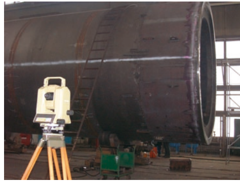
Figure 2b. A side view of the crane column in the assembly hall.
