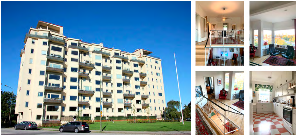
Figure 1. Exterior and interior of Peterstorp (photo from www.hsb.se and private tenant).
