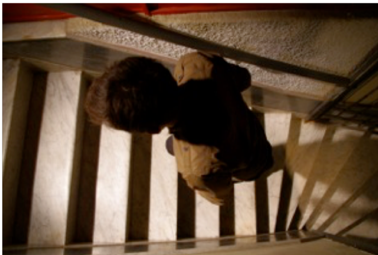
Figure 3: Staircase of the school building (Researcher's archive)
