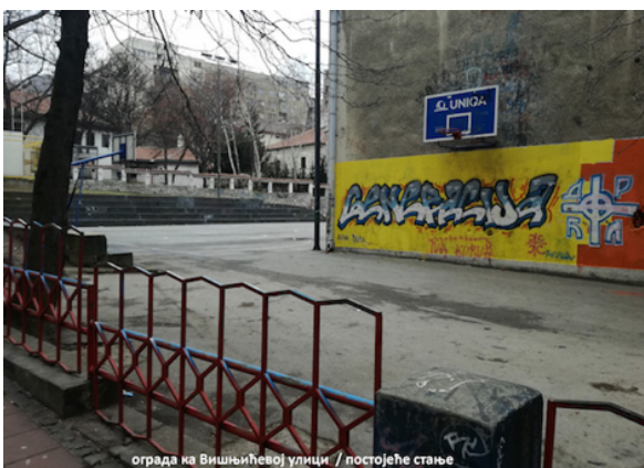
Figure 12: Fence, actual state.
