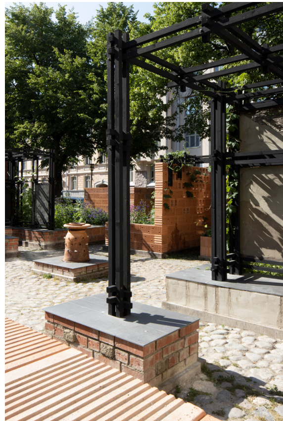
Figure 10: Clay in different forms was used in the construction of the space. The terracotta-colored elements are fired clay, and the grey ones are raw unfired clay. The raw clay bricks contain reed that comes to surface as the structure erodes. The clay plastered elements on the pergola change their appearance as erosion progresses. Alusta Pavilion. June 2023. Photo: Maiju Suomi.
