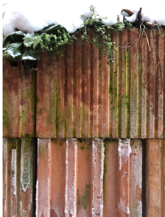
Figure 14 (right): Fired clay blocks with algae and frost on them. Alusta pavilion. November 2022. Photo: Elina Koivisto.
