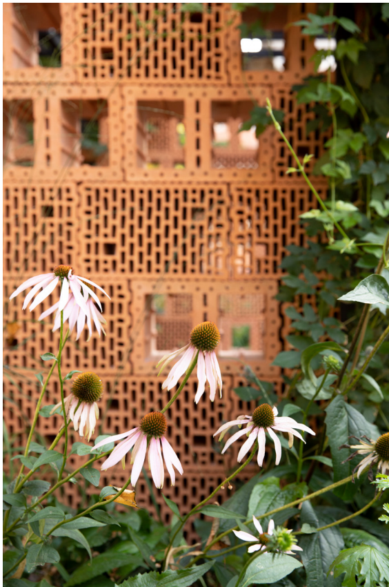
Figure 8 (left): Porous clay blocks. Common Hops ( Humulus lupulus ) and Purple Coneflower ( Echinacea purpurea ). Alusta Pavilion. August 2022. Photo: Maiju Suomi.
