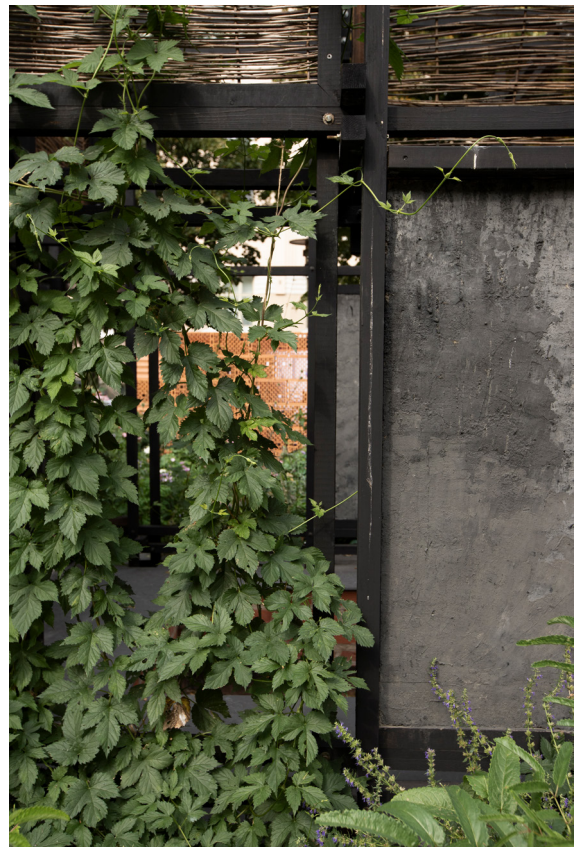
Figure 3: Wooden pergola with panels of woven wicker, partly rendered with mortar made of biochar and raw clay, subject to alteration through erosion. Common Hops ( Humulus lupulus ) rising to cover the openings of the pergola. Hyssop ( Hyssopus officinalis ) and Great Burnet ( Sanguisorba officinalis ) growing in front. Alusta Pavilion. August 2022. Photo: Maiju Suomi.
