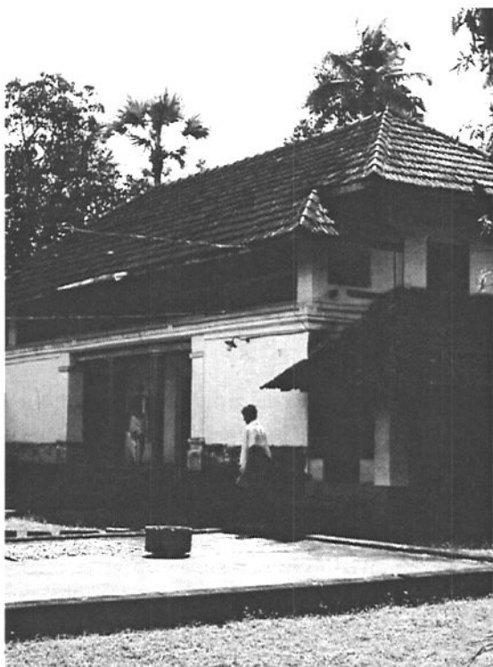
Fig. 23. Nellikāṭṭu Māmaṅṅu Mana: the main building. Photo MP 1983.
