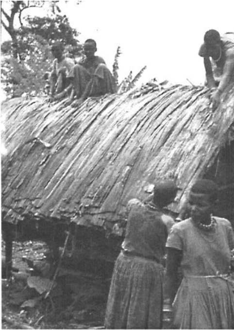
Fig. 14. Roofs of houses and storehouses are usually made and repaired in cooperation with neighbours (P 76).
