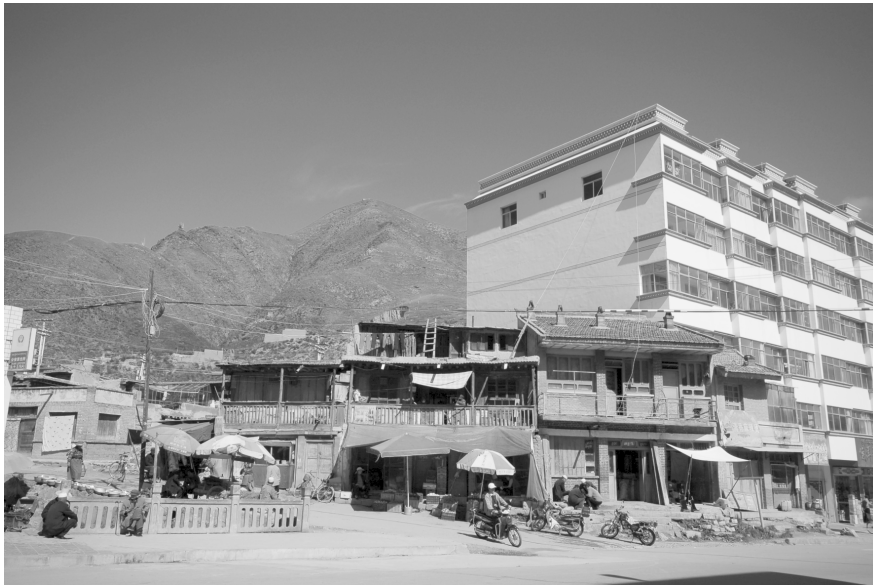
Figure 1 On the threshold of changes: old shop houses and a new block along the main street in Xiahe in 2007.
