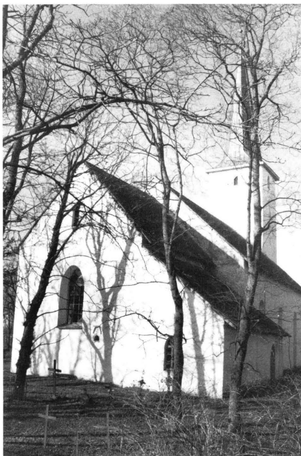
Fig. 11. The Church of Viru-Nigula seen from the northeast. The sacristy with its sloping roof was built after the chancel was completed. The sacrament opening can be seen on the north side of the window in the chancel wall. — Photo MH 31. 3. 1990.
