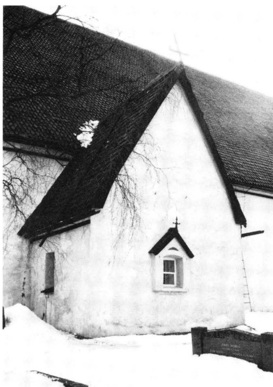
Fig. 9. The Church of Pernaja, the sacristy seen from the northeast. — Photo MH 24.1.1991.
