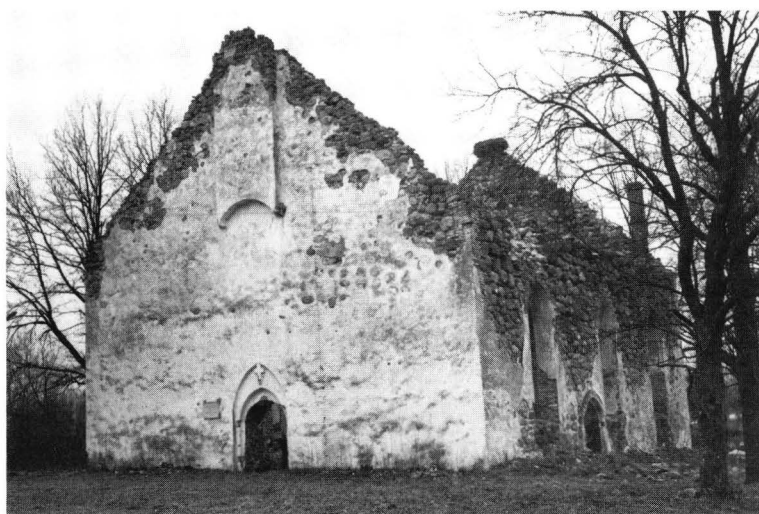
Fig. 22. Ruins of the Church of Rannu, southwest view. The lower part of the console tower is visible in the west gable end. The church was destroyed by Soviet artillery fire in the spring of 1944. — Photo MH 28.3.1990.
