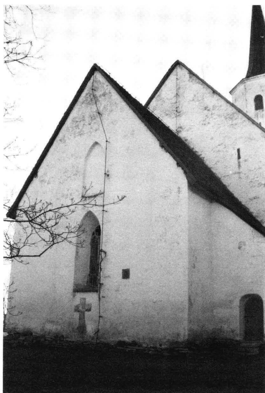
Fig. 15. The Church of Haljala, the chancel seen from the southeast. The chancel was built after the nave was completed. There is a limestone cross below the chancel window; similar crosses in corresponding locations are in the Churches of Korpoo and Vehkalahti in Finland. — Photo MH 31.3.1990.
