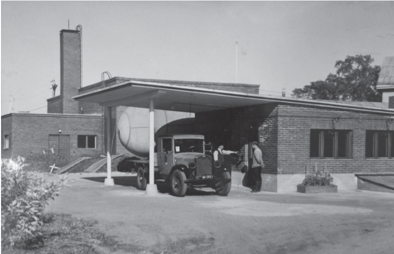
Figure 8. Ford truck filling biogas at a CBG filling station at Rajasaari Sewage treatment plant in Helsinki in 1943. Photo: Foto Roos/Photo archive of Helsinki City museum.
