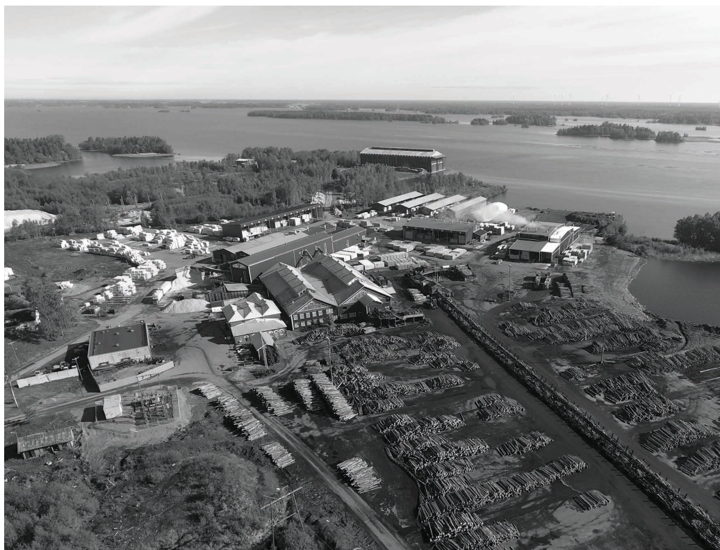
The industrial area of the Pihlava Sawmill in summer 2017. The log field and the log board have replaced the log pond and the former transporter. Over recent decades several additions have been added on. Photo: Jussi Miikkulainen, 2017.
