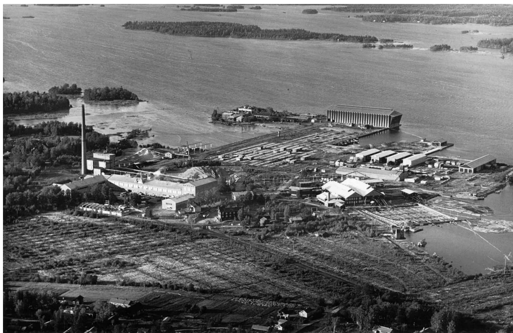
The Pihlava Works area in the early 1960s. The fibreboard factory is on the left and the power station behind it. The sawmill and the log pond appear on the right. The huge timber-framed shed is on the coast. As the sawn timber was kiln-dried, the former piles disappeared from the industrial landscape and only the traces of the stacks can be seen on the ground. Photo: SKOy.
