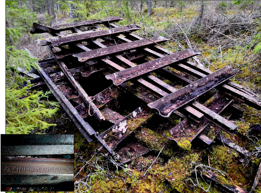
Figure 7. Tracks and other parts of the original Hyrynsalmi-Kuusamo railroad found in the wilderness, and now being re-used for building a private narrow track railroad by a Finnish railroad enthusiast Leo Saha. Inset: Krupp factory stamp on one of the tracks. (Photographs: Leo Saha.)
