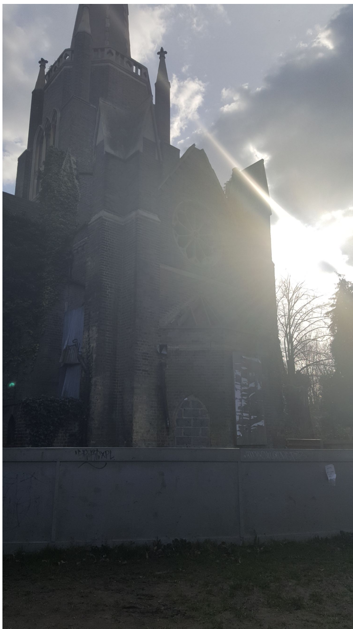
Photo 5. Abney centre chapel in partially ruinous state. Photo: Romany Reagan, 2015.
